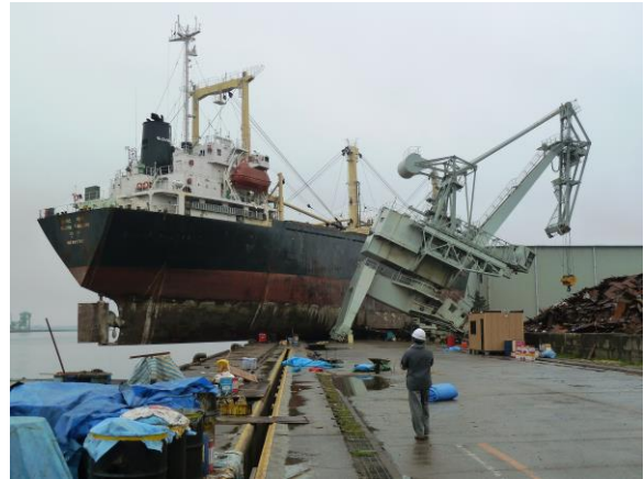
Ship impact with crane and warehouse, Sendai, Japan
